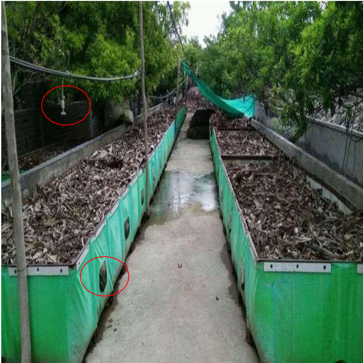
Photograph of Composting facility
