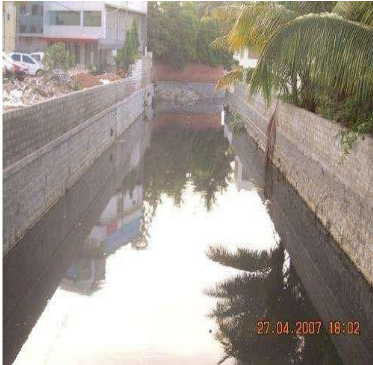
Photograph of SWD with no visible/floating solids
