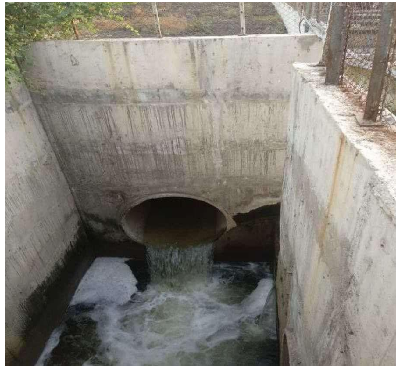
Photograph of outlet treated wastewater
