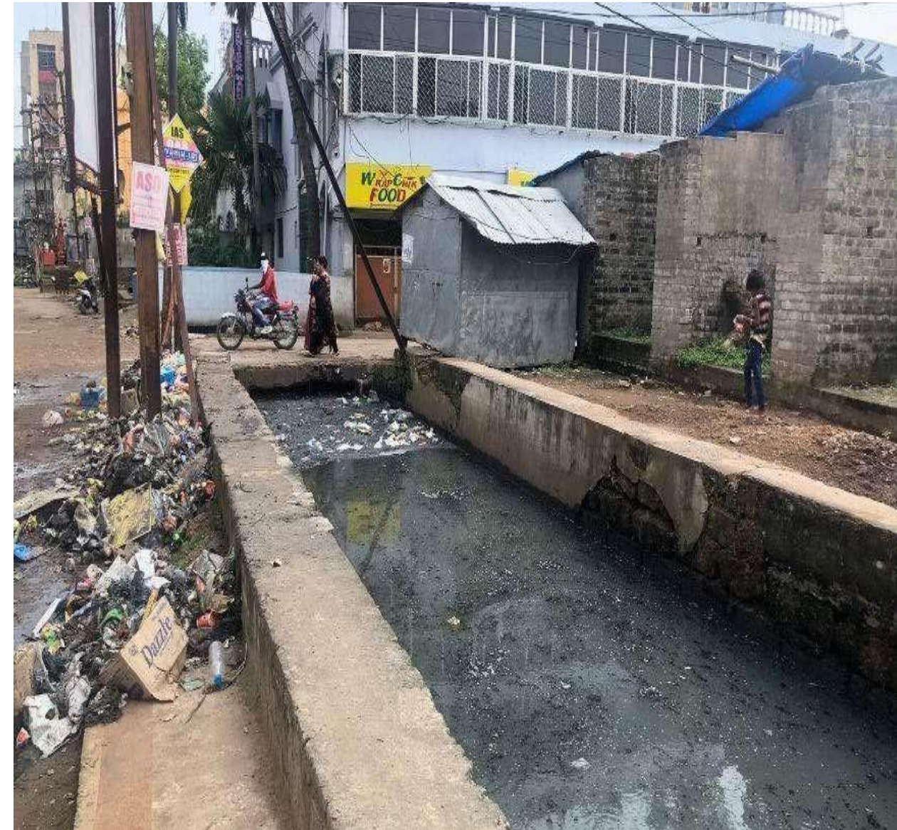
Photograph of SWD with visible/floating solids
